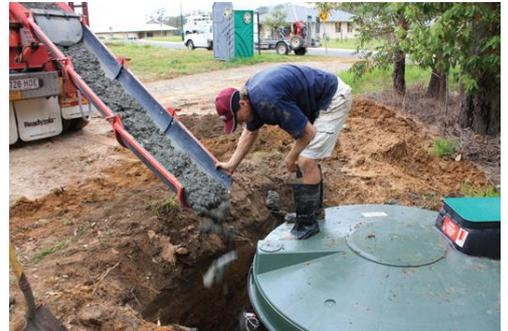
19. Before concrete is poured, the tank must be filled with 900 litres of water. This provides weight to prevent movement of the tank when the concrete is poured
